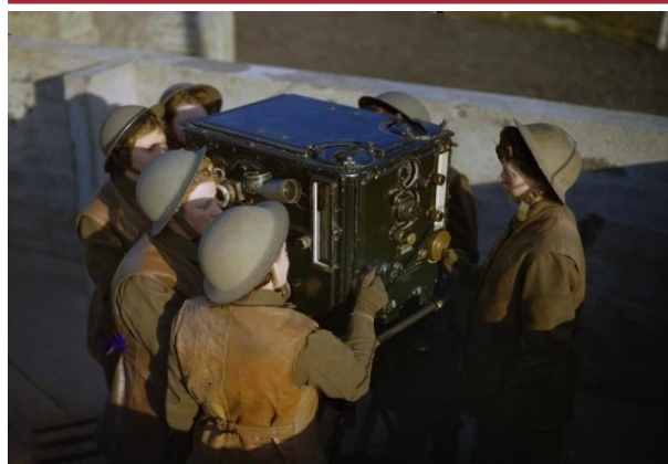
ATS crews "man" the optical rangefinder (above) and the mechanical range computer (below). The firing solution was fed to the gunners on dials and manually matched.
