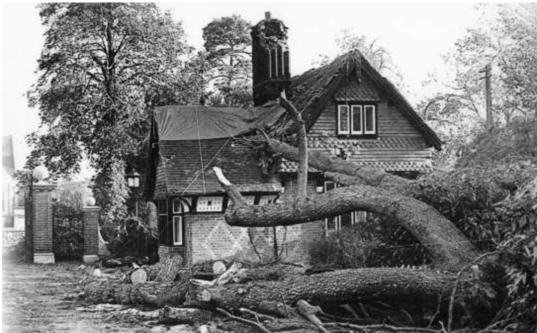
A typical Kent peg tiled house damaged by a fallen tree during the hurricane of 1987
